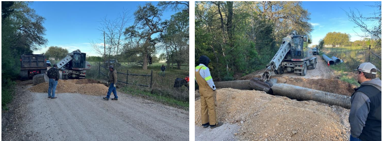
Figure 25 – Dannheim Road Culvert Replacement 3/17/2026
