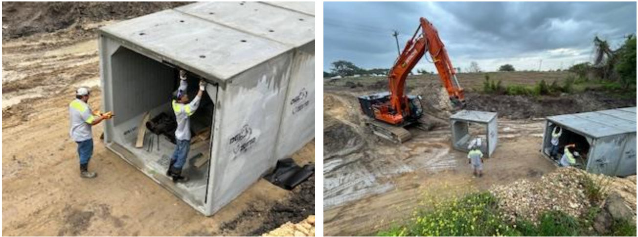
Figure 20 - Reinforced Concrete Box Culvert Install on Old Independence Road 4/2/2026
