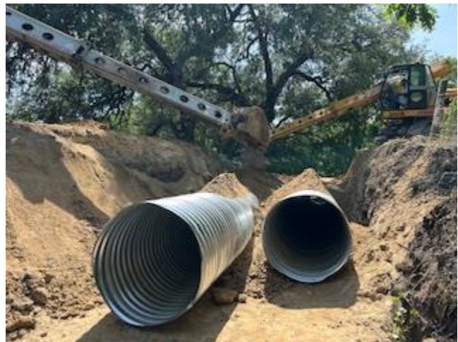
Figure 22 - Quebe Road Culvert Replacement 4/18/2026
