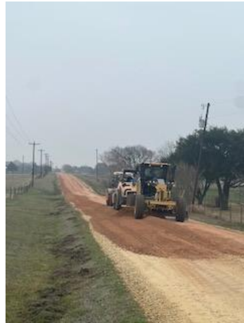
Figure 13 – Zibilski Road Base Installation 2/23/2026
