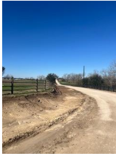
Figure 10 – Egypt Road Ditching and Road Widening 3/3/2026
