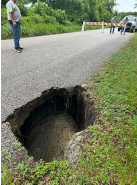
Figure 23 - Quebe Road Culvert Failure 6/12/2025
