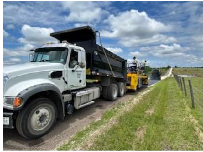
Figure 15 – Whitman Road Chip Seal Application 5/11/2026
