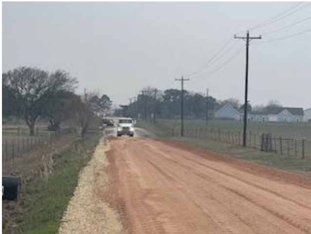
Figure 12 – Maass Road Base Installation 2/19/2026
