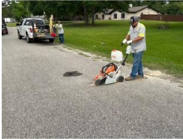
Figure 26 – Live Oak Drive saw cutting in preparation for the culvert replacement. 5/18/2026
