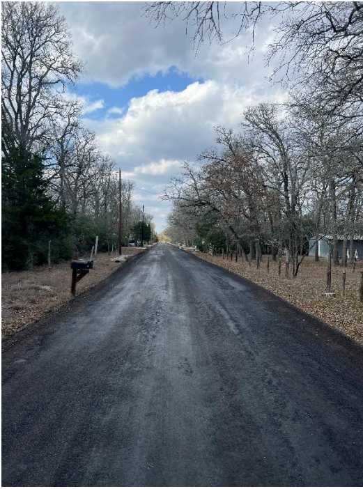
Figure 14 - Edgewater RAP Installation – 2/12/2026
