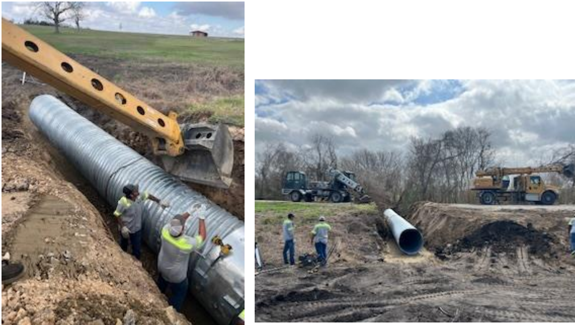
Figure 24 - Bosse Road Culvert Installation 3/5/2026
