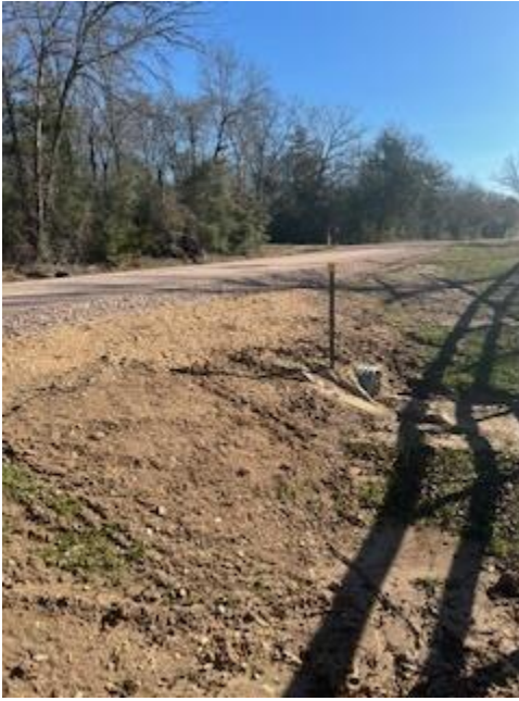
Figure 11 – Dove Lane Culvert Replacement and Base Installation 1/13/2026
