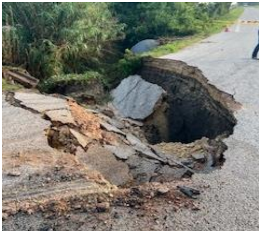
Figure 19 – Old Independence Road 2025 Culvert Damage 6/5/2025
